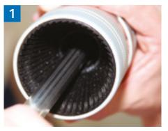
Cut the pipe to length and deburr inside and out so as not to damage the seal ring. Clean chips from the pipe end.
