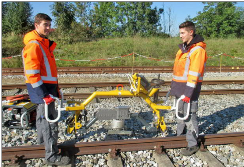
Fig. 35: Put the machine on the rail
