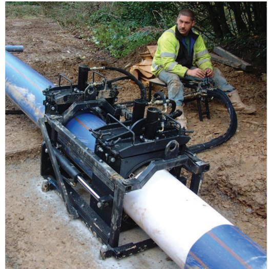
The 355 (Left) and 500 (Right) Hydraulic Pushing Machines on site inserting sticks of PE pipe
