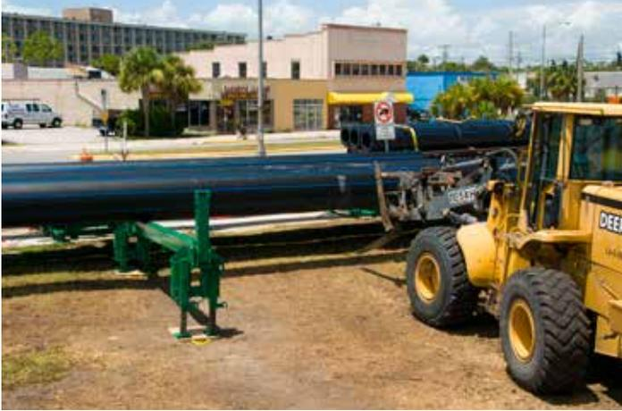
Pipe can be loaded directly from the truck onto the racks.
