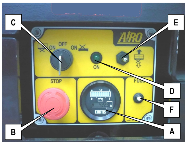
5-3: Ground control panel
