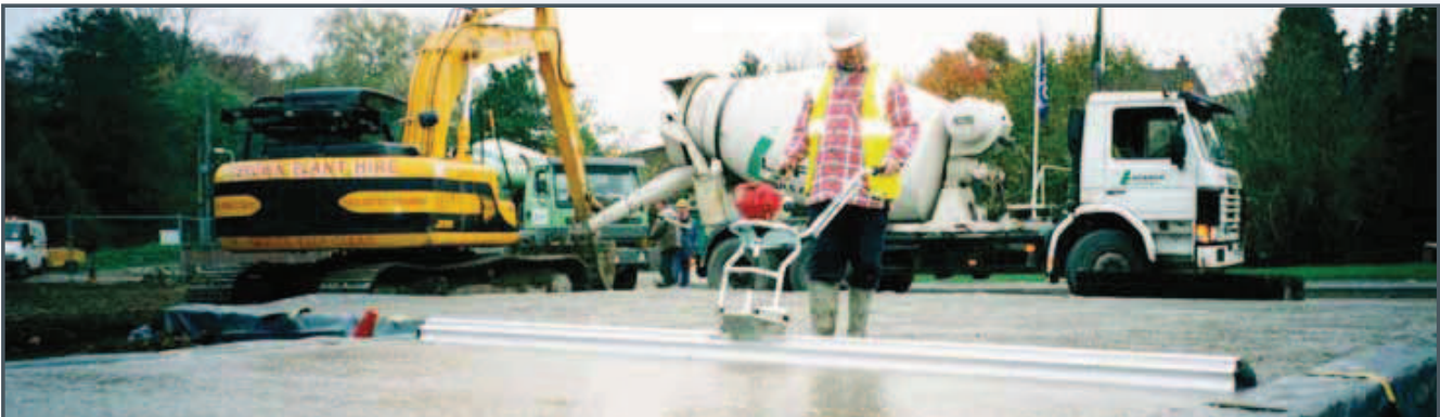
Simple one-man operation, even on large bays of concrete
